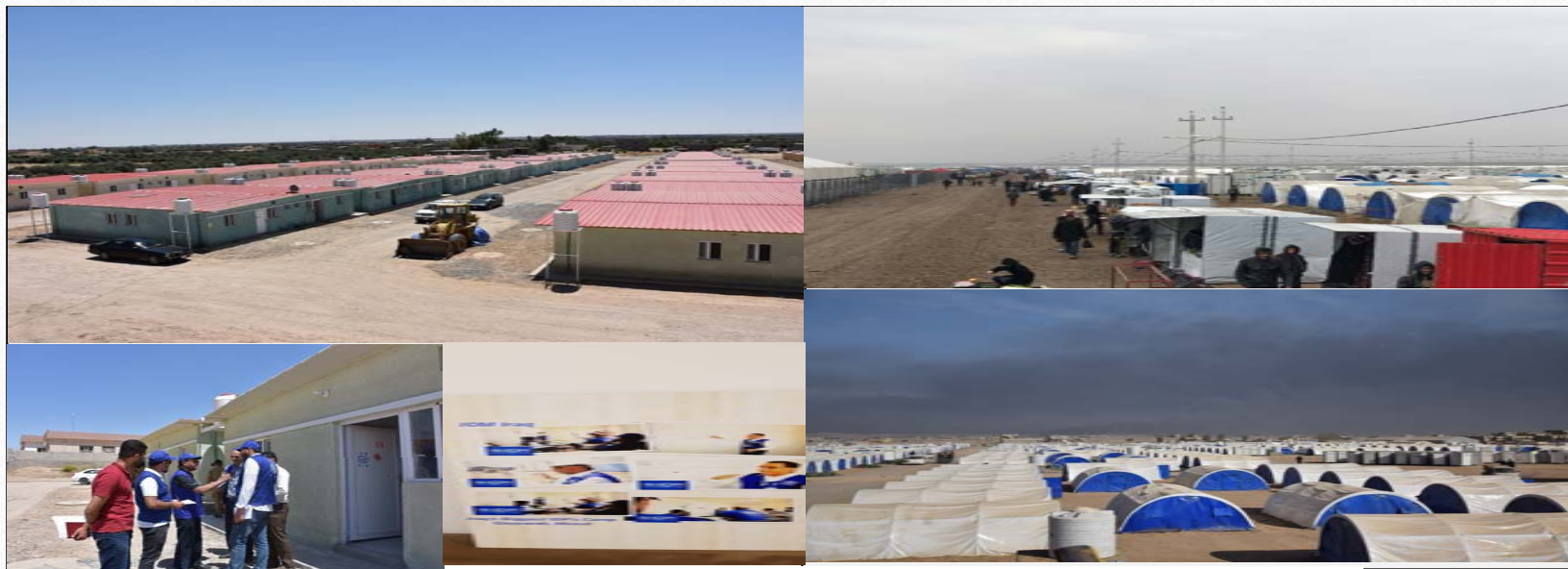
Shelter Housing and IDP Emergency Camp Projects
